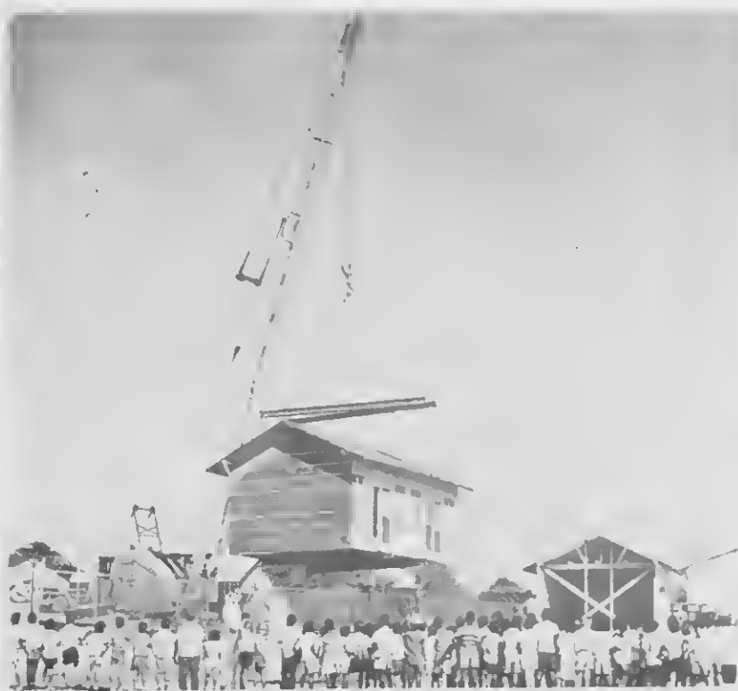
FASCINATED STUDENTS of St. Augustinus College watch as a crane lifts a former Lago bunk house over the fence. A gift from the company, the building will be used by the school for special purposes.
